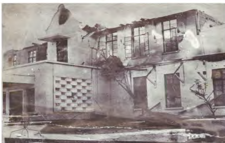
The official residence of the late Sardauna completely gutted by fire following the shelling on the building by the coupists
