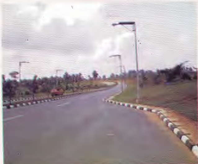
Solar Street Lighting in Uyo, Cross River State
