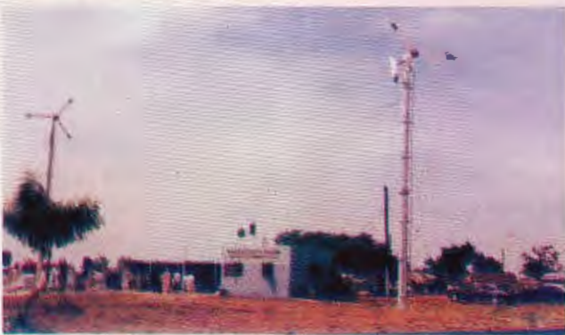
5kW aero generator in Sayya Gidan Gada, Sokoto State
